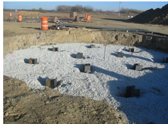
Driven piles before concrete cap is poured
