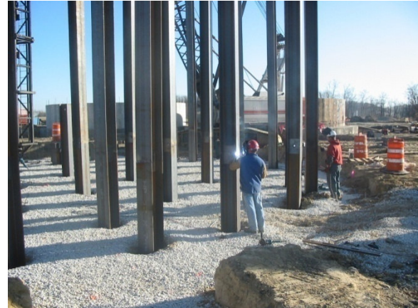
50 ft. H-Beam being spliced to 70 ft. H-Beam
