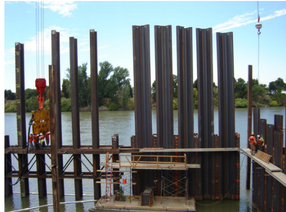
Steel sheet pile being driven for Combi-Wall
