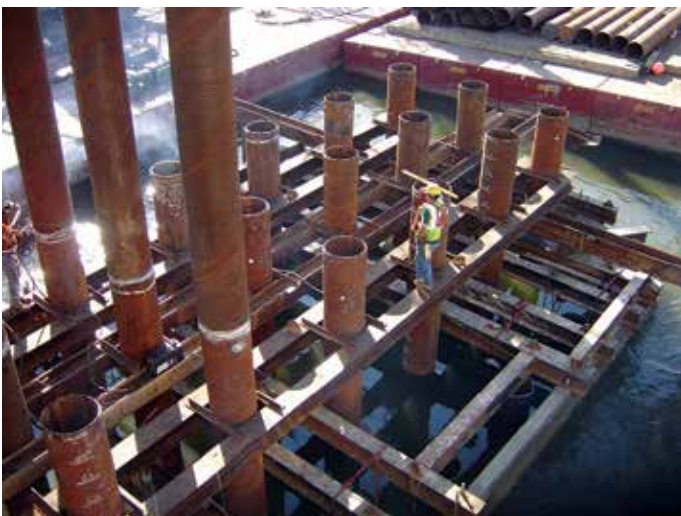
Route 70 Bridge over the Manasquan River, Brielle, NJ
