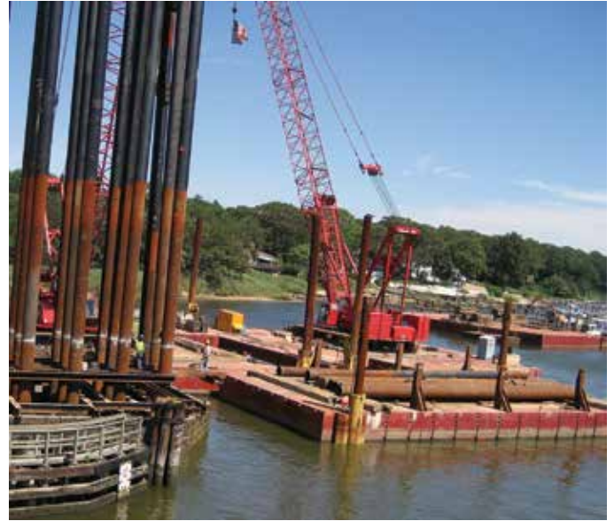
New Jersey Department of Transportation, Brielle, NJ
